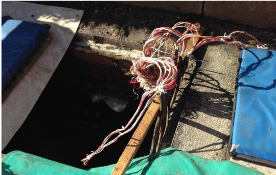
Figure 1 Copper wires in a UK manhole under repair
